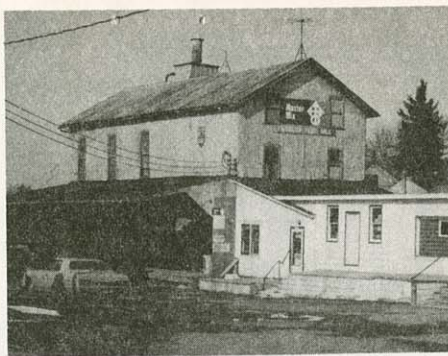
Fessler's Feed Mill and Elevator. Elevator built in 1901.
